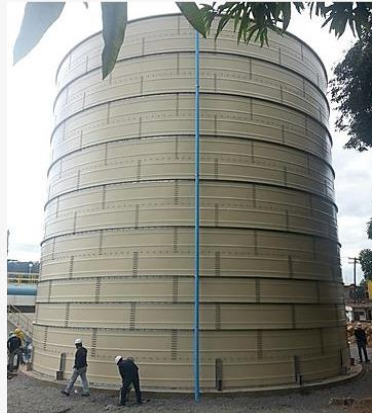
2000 cum capacity, 14m diameter x 13.48m height steel bolted tank. The biggest in the Philippines.
