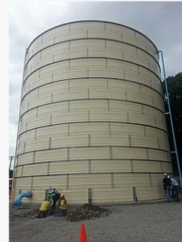
2000 cum capacity, 14m diameter x 13.48m height steel bolted tank. The biggest in the Philippines.
