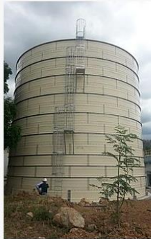
2000 cum capacity, 14m diameter x 13.48m height steel bolted tank. The biggest in the Philippines.
